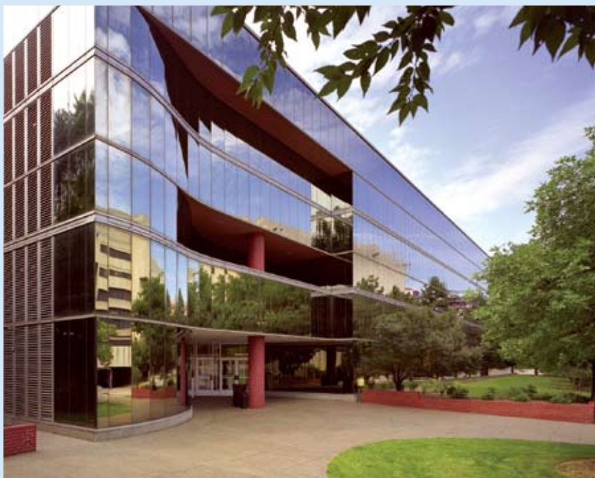
Internal renovations at Mervis Hall continue as part of a long-term improvement plan.
